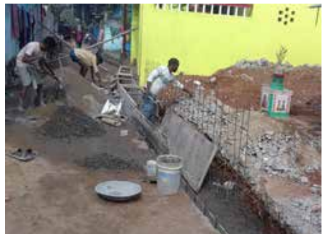
Drain being built as a result of children's collective action
